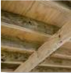
12" On-Center Floor Joists
