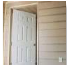
Interior Wall (Cottage)
